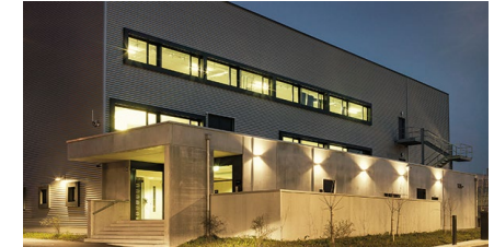
Equinix ZH5 IBX exterior
